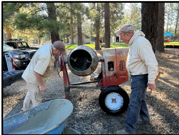
Pouring concrete footings: Tom Nixon (right) and Greg Zirbel.
